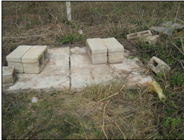
Figure 3-24 Concrete lined pit for sharps disposal at a Clinic
