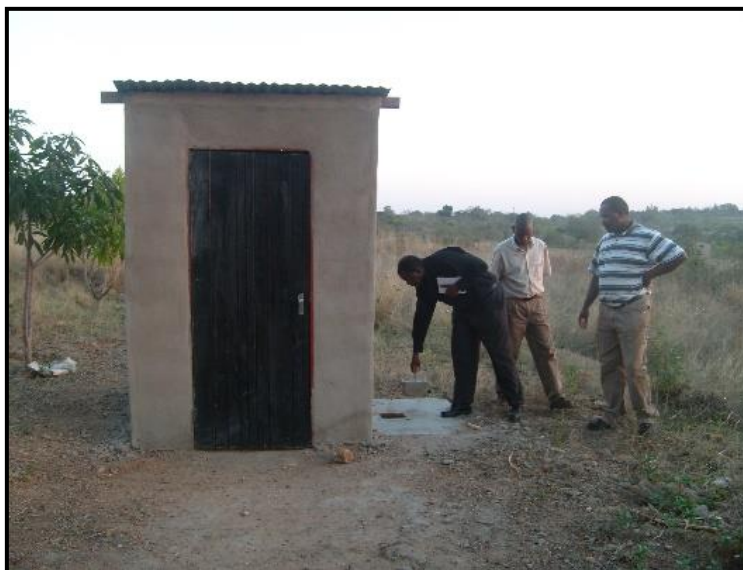
Figure 3-25 Concrete lined pit for Home based Health Care Waste
