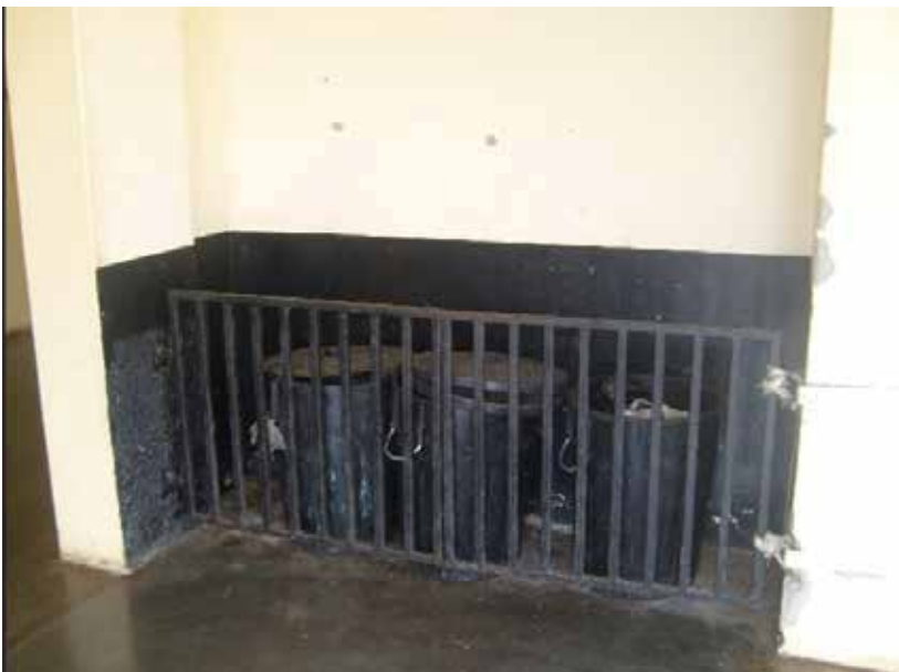
Figure 3-18 Temporary storage for waste
