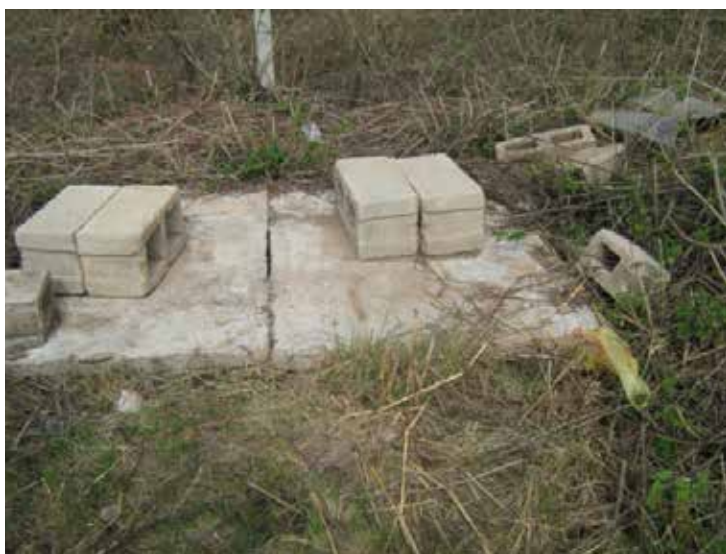
Figure 3-21 Concrete lined pit for sharps disposal at a Clinic
